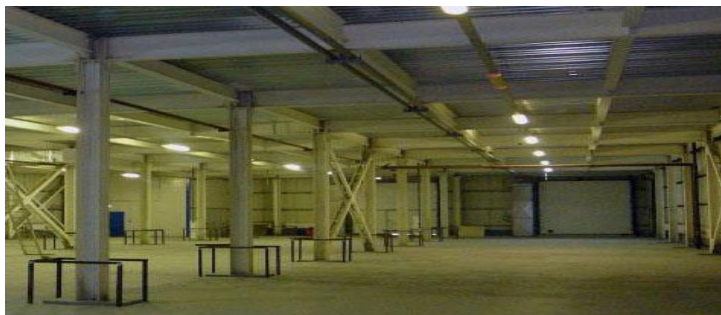
Photo 2. Category B warehouse
